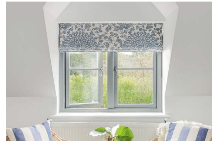
Right The interior finish of these painted softwood double casement windows is Teknos grey. The windows are fitted with glazing bars and monkey tail window fasteners.
