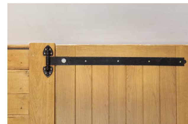
The long straps of the hinges are required to hold garage doors because of their size and weight
