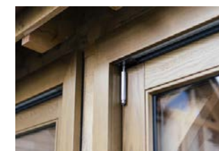
Left These doors have 3 pairs of satin chrome hinges.
