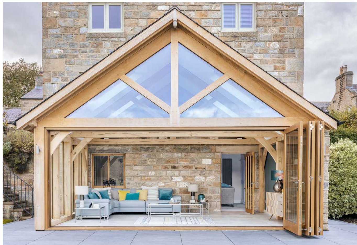
Above These open bifold doors concertina neatly to form five equal panels, hung in a 5R (five right) lay out.
