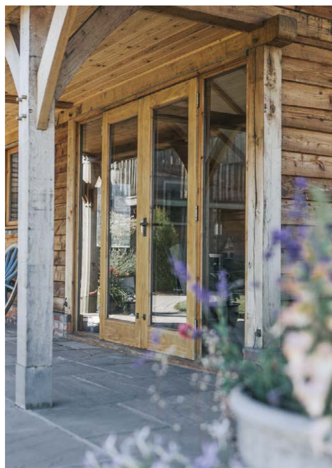
Left These French doors are accompanied by a fixed screen on either side to maximise light into the room. During the design stage of your project you will work with your Design Consultant to select the features you would like in your doorway.
