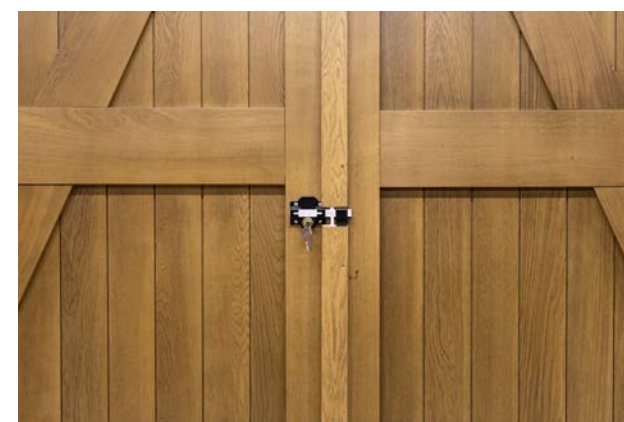
The through bolt from the inside
