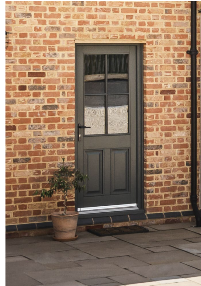
Above This personnel door is half glazed with vertical and horizontal glazing bars.
