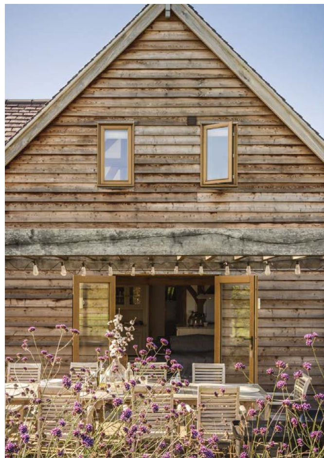
Left These two single casement windows on the weatherboarded gable-end have a Teknos coating guaranteed for 5 years. They are both hung on the left side.
